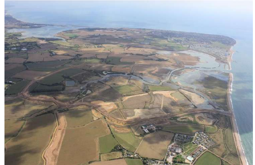
Medmerry Managed Realignment Scheme
