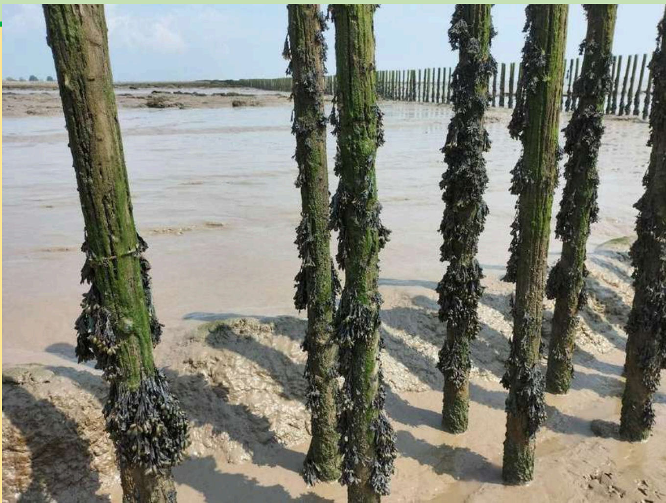
Derelict fenceposts – note scour at base of posts
